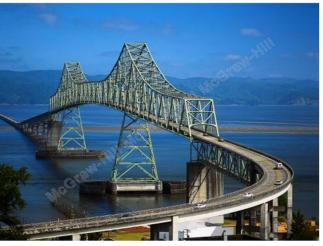
Calculate the force in each member of this structure (a truss) in order to design it to withstand the loads that it will experience.
